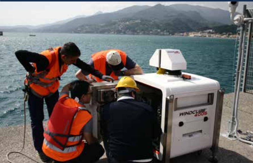
LIDAR SCANNER WINDCUBE 400S IN THE PORT OF VOLTRI, GENOVA
